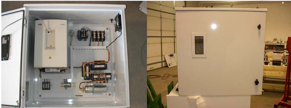
15 hp drive with harmonic filter
